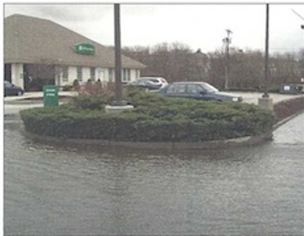
Water roared through the Mendon Road branch parking lot in Cumberland RI, turning the branch into an island, undamaged inside by water.
